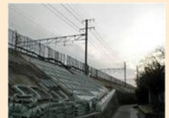
Landside prevention measures
