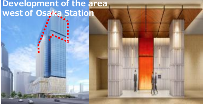
(Left): Upper floors 30 to 38 are hotel guest room floors. (Right): Illustration of the hotel front entrance (1st floor)
