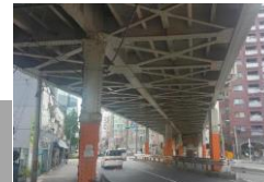
Steel bridge piers
