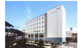
JR Takatsuki NK Building (Opened in June, 2009)
