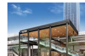
Bentencho Station remodeling
