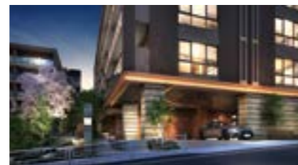
Predear Yokohama Yamate Park Villa (to be completed in August 2023)
