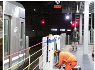
Platform barrier installation work
