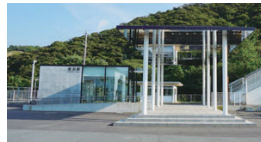
Higashi-hama Station is a ZES pilot station
