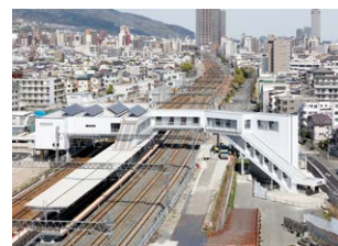
Various energy-saving features installed at Maya Station
