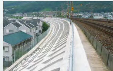
Slope reinforcement and other disaster mitigation measures have been implemented
