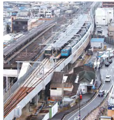
February 2015 Services commenced first on the Wakayama-bound elevated platform and tracks at Higashi-Kishiwada Station on the Hanwa Line
