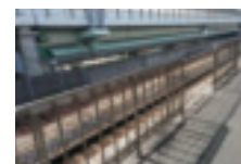
Platform fence for bypass lines
