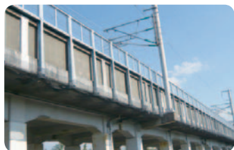
Noise barriers installed alongside Shinkansen rail lines
