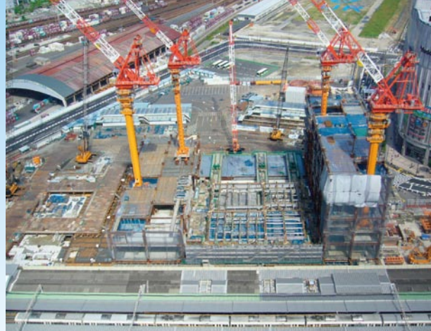
The New North Building under construction
