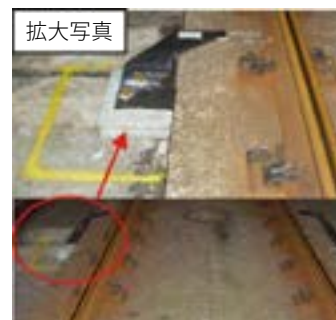
写真3：補修構造の敷設状態
