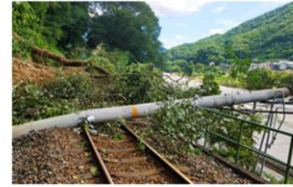
Hakubi Line (Bitchu-Takahashi Station - Kinoyama Station segment) concrete pillar snapped, soil eroded
