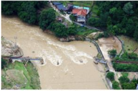
Geibi Line (Shirakiyama Station - Karuga Station segment) No. 1 Misasa River bridge girder wash away
