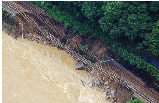
Sanyo Line (Hongo Station - Kochi Station segment) flooded
