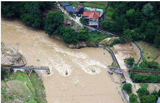
Geibi Line (Shirakiyama Station – Karuga Station Segment) No. 1 Misasa River bridge girder wash away
