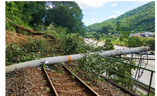
Hakubi Line (Bitchu-Takahashi Station - Kinoyama Station segment) concrete pillar snapped, soil eroded
