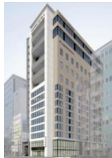
Hiroshima Hacchobori NK Building
