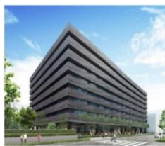
Osaka Kita NK Building
