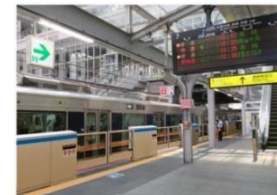
Installing platform gates at Osaka Station (platforms 6 and 7) (representative image)
