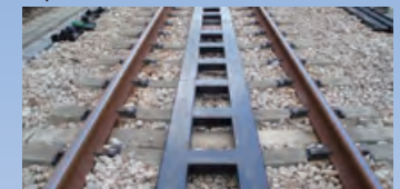
Derailment prevention guard
