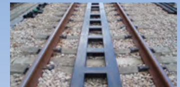
Derailment prevention guard
