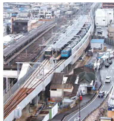
February 2015 Services commenced first on the Wakayama-bound elevated platform and tracks at Higashi-Kishiwada Station on the Hanwa Line
