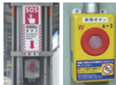
Platform emergency button (Left) For Shinkansen station (Right) For conventional line station
