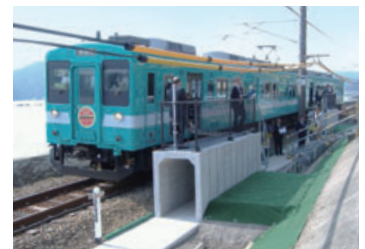
Train exit platform for evacuating from trains at locations between stations
