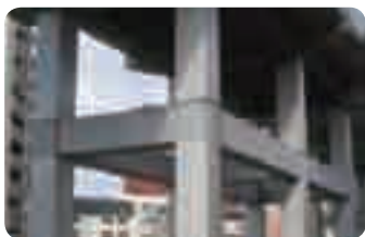
Elevated railway tracks with reinforced earthquake resistance
